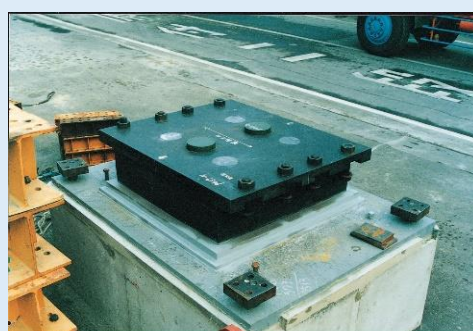
⑥ 免震支承
